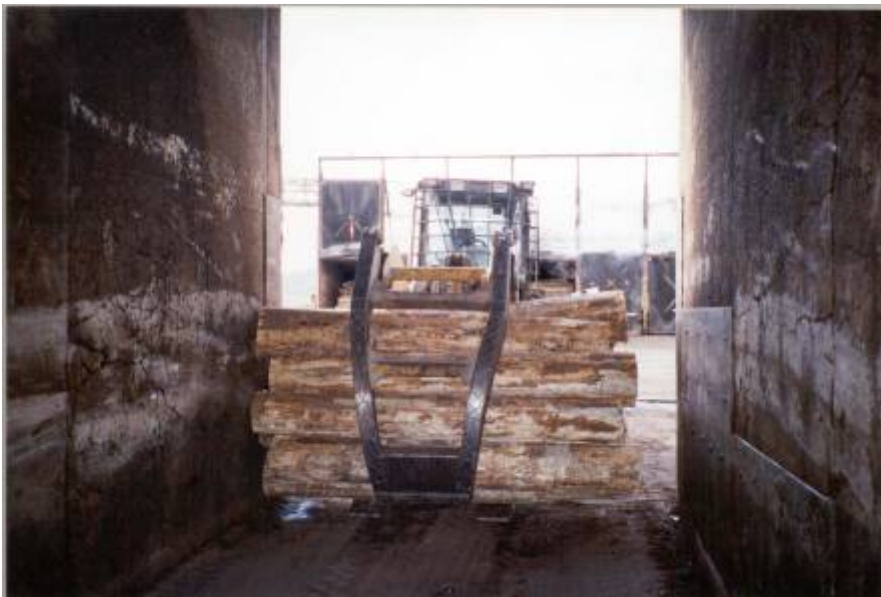
Figure 2: This photo demonstrates the typical clearance from the tunnel walls when a log loader places peeler logs in a vat.
